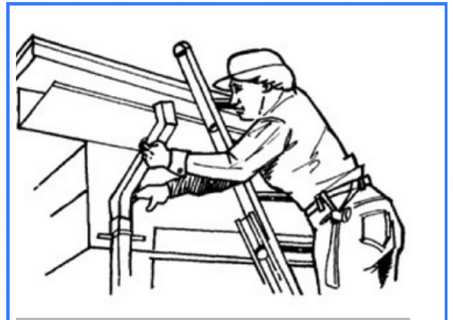
REMOVE DOWNSPOUTS/TIE BACK SHRUBS
