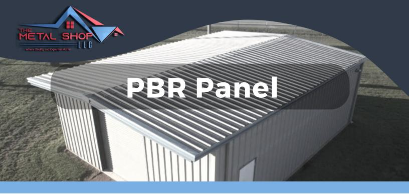
"PBR" stands for "Purlin Bearing Rib" panels. This means that the panels have a larger overlap section that completely overlaps the next panel. This creates more metal to metal contact which yields a stronger connection and more weather-tight metal roof panels.
